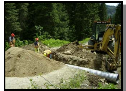
Above are (L to R) Jean Neigum, Kim Marshall (Curly) & Caitlin Dobson, QA at the Rip Rap site on Hwy 3. Below Lynn Davey, Garry Campbell & Dave Johnson do a culvert install on the Paulson Detour
