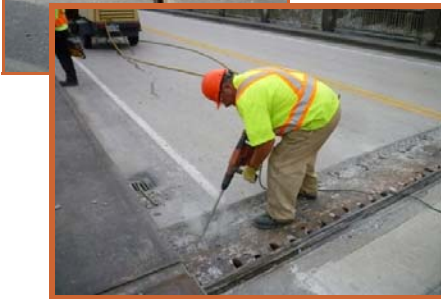
On the left —Rob Konkin chipping concrete at Brilliant Bridge.
