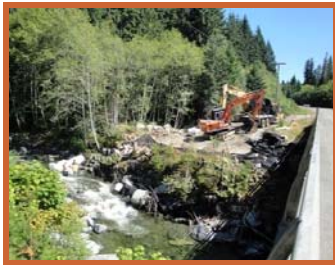
Bridge crew installing berms and fish catchment nets in creek.
