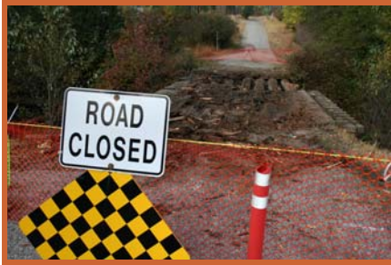
A picture of the Louisa Street Bridge when it was closed
