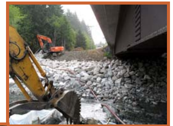
Above—Deflections Berms Below—Working under the bridge
