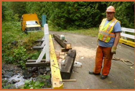
On the left—James Kastrukoff replacing posts on IXL Bridge near Rosslund.
