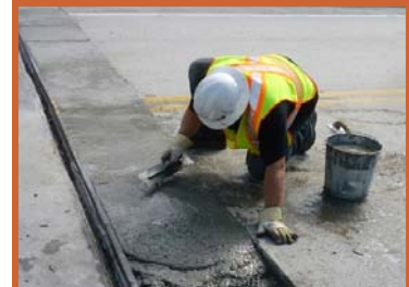
On the right—Mike Prystae trowelling concrete at the Brilliant Bridge in Castlegar.
