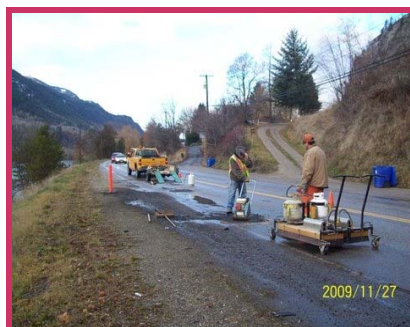
Birchbank Road Crew Ray Wilson & Mark Tomasini Patching on Hwy 22
